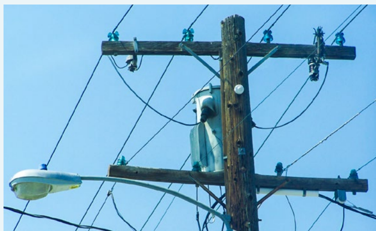
CD 257 Mickeys and CD 252 Hemingray No 2 Cables on top Cross Arm CD 162 No 19 on Bottom Cross Arm which is a 4 KV Circuit from Butte MT Photo by Justin Martin
